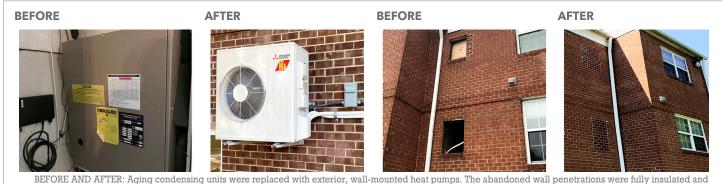
BEFORE AND AFTER: Aging condensing units were replaced with exterior, wall-mounted heat pumps. The abandoned wall penetrations were fully insulated and finished with brick.
